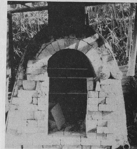
Their old kiln which was made at home & called Catenary Arch.
